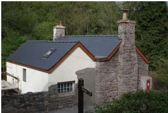
Fig.70 Manor Brook Cottage new extension
