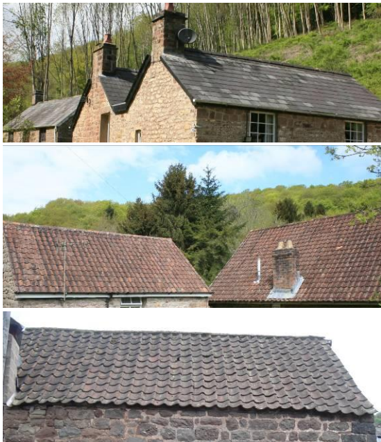
Fig.79 Characteristic roofing materials: Natural slate and clay pantiles
