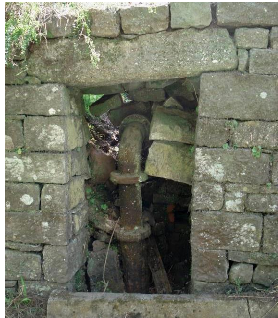
Fig.31 Historic iron pipe taking water from Manor Brook under the road to Clearwater Mill
