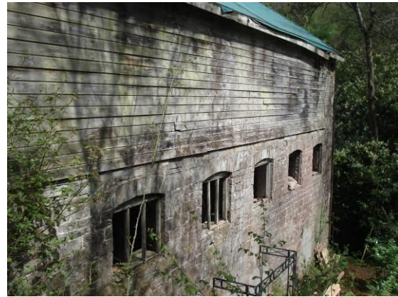
Fig.50 The east facing elevation of Fernside Mill
