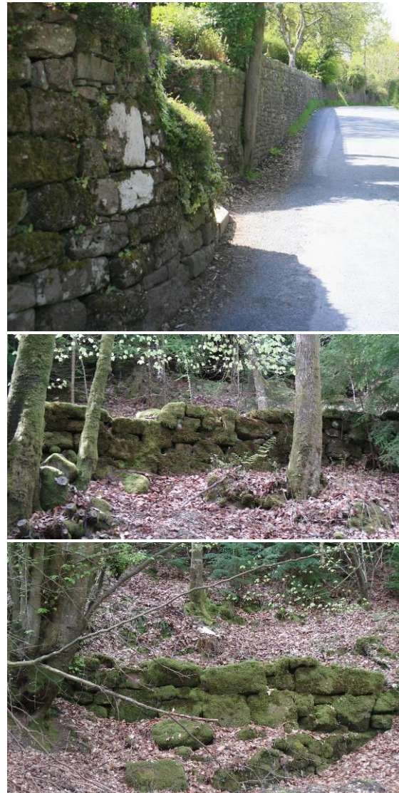
Fig.80 Typical stretches of boundary walls
