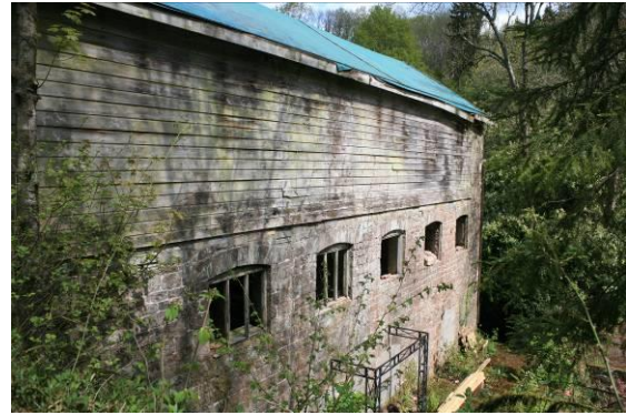
Fig.35 Fernside Mill from the east side
