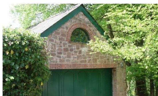
Fig.76 Rubblestone is even used in modern additions such as this garage
