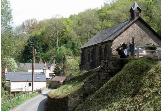
Fig.13 A grouping of buildings including the Old Trinity Church, Manor Brook Cottage, the Bell and outbuildings seen here
