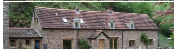
Fig.26 (right) Materials found in the character area. From top: Clay pantiles, white-washed rubblestone with natural slate and stone stacks, quartz conglomerate rubblestone with Bridgewater tiles.
