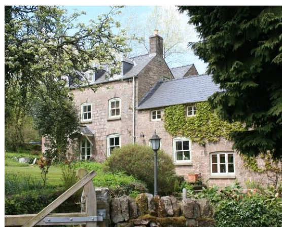
Fig.33 The double-pile New Mills Farm with dormers in the attic
