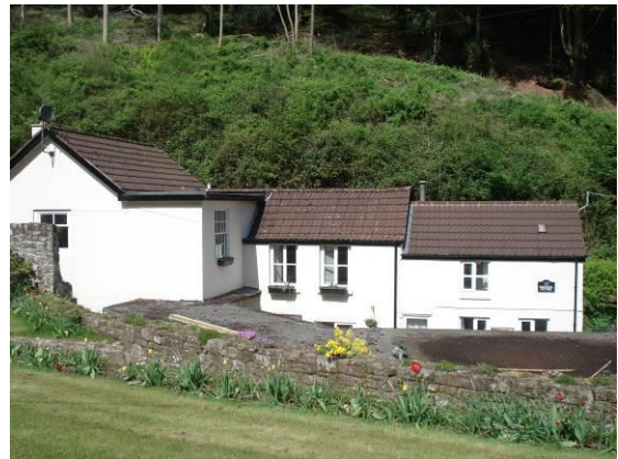
Fig.72 The heavily altered Fern Bank
