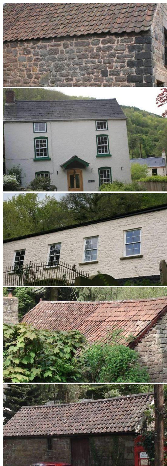
Fig.17 Materials found in the character area. From top: Slag blocks used in conjunction with quartz conglomerate rubblestone, smooth render and natural slate roofs, white-washed rubblestone, Bridgewater tiles, pantiles
