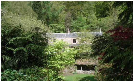
Fig.27 Glimpsed view of Traligael from the road
