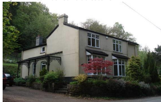
Fig.78 Smooth render painted cream at Woodside (probably a remodelling of an exposed stone cottage)
