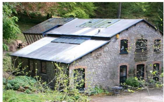
Fig.74 The Coach House with extension to rear
